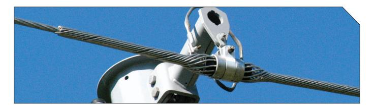
The Fiberlign Suspension provides superior cable and fibre protection at the support point. The combination of structural reinforcing rods, outer rods, 'boltless' housing and resilient inserts reduces compression, clamping, and bending stresses on cable. Negative effects of wind-induced cable motion, such as aeolian vibration, galloping, and wind sway are also minimised.
